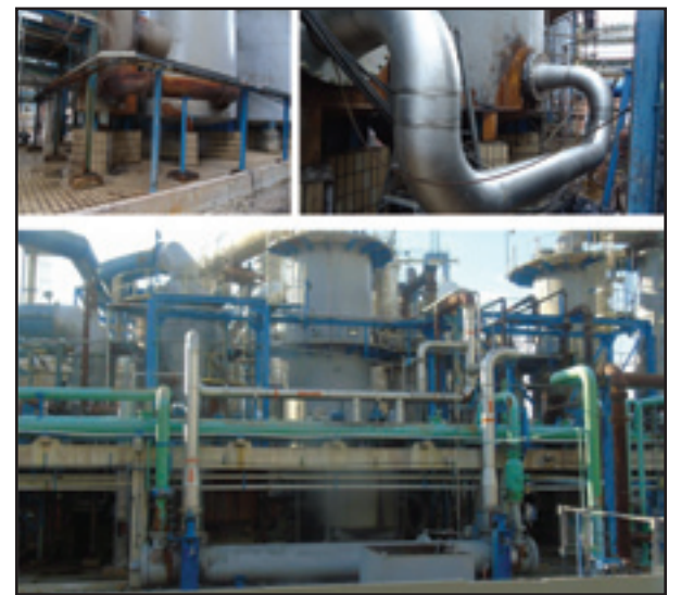
Cast iron piping replacement with CSX™ HSSS (Elekeiroz, 2020).
